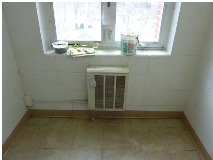
Typical electric heater at each end of corridor is shown to be replaced in Year 1.
