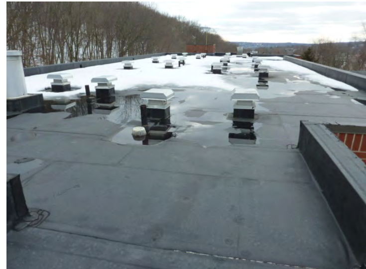
EPDM roofing membrane installed in 2002.
