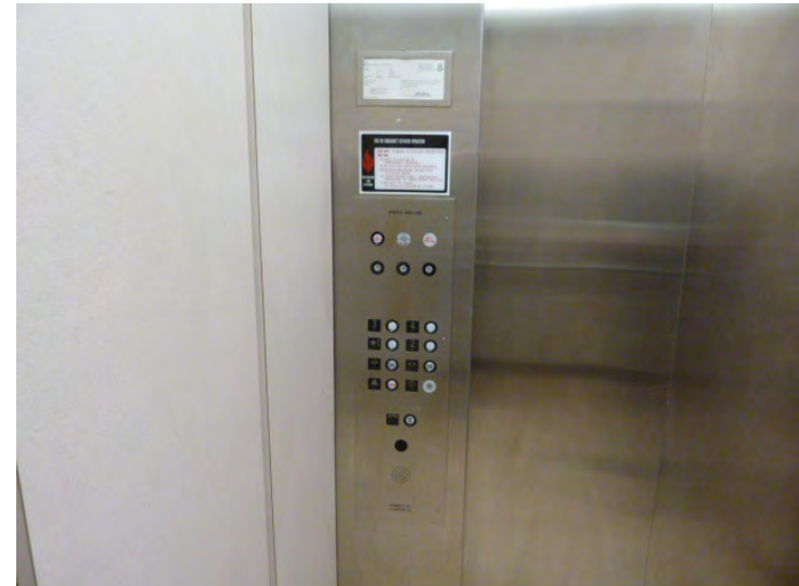
The accessible elevator cab is the proper dimensions and the control panel is at the proper height.
