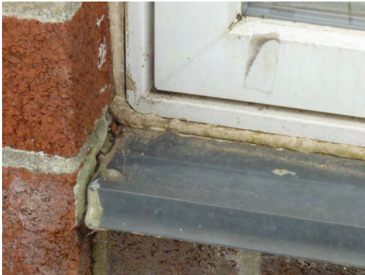
Typical open joints at window sills.
