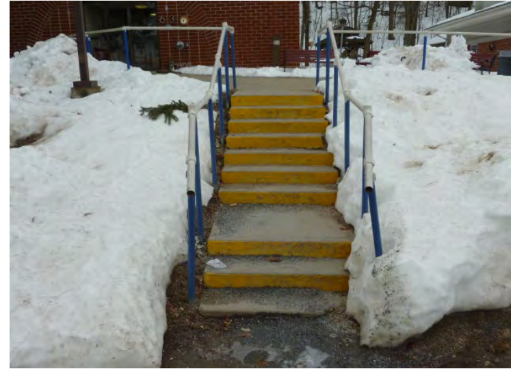
Typical concrete walk and rail are in poor condition.
