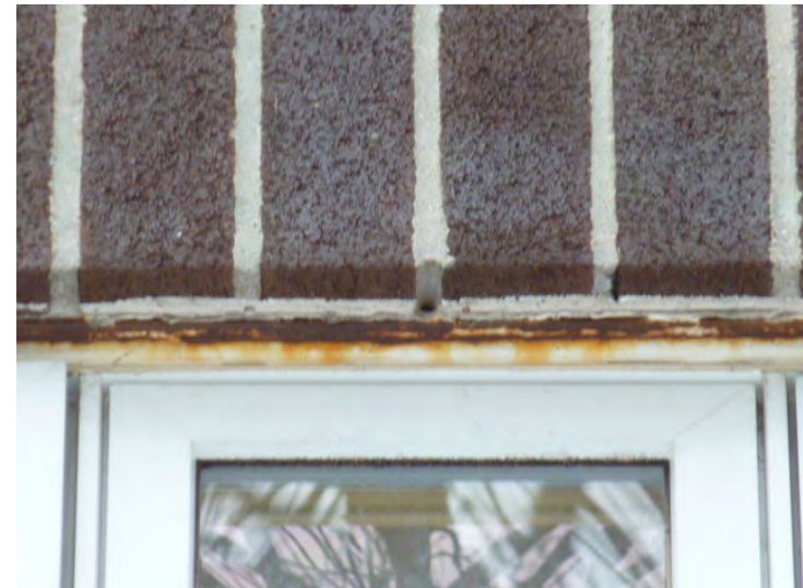
Typical rusted lintel at window head indicating a flashing failure building wide.
